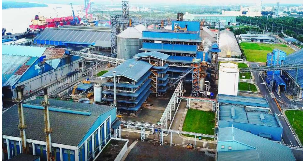
Stabilization – Extraction – Neutralization Plants Complex
